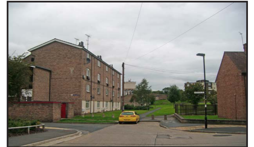
1960s estate - Howe Hill, with water tower visible in background
