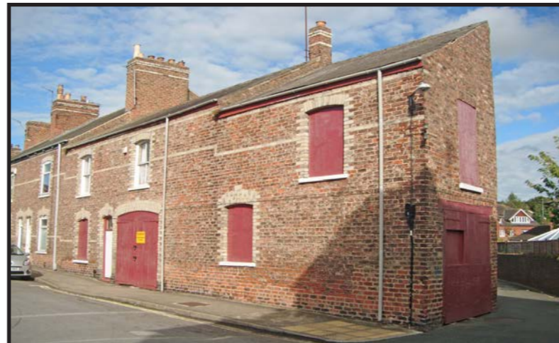
Old loading building in Acomb Terraces
