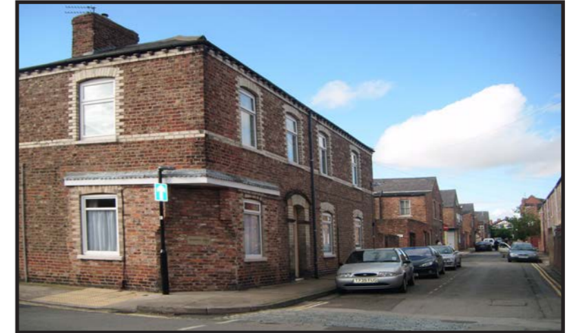
Ex-corner shop and patch of stable pavings on School Street
