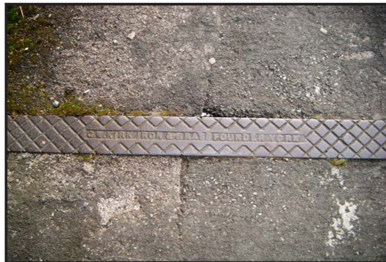
Drain cover, Murray Street
