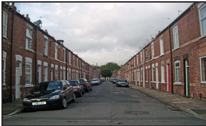
Example of terraced street in Leeman Road area
