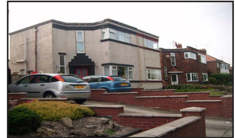
1930s Art Deco buildings on Salisbury Road
