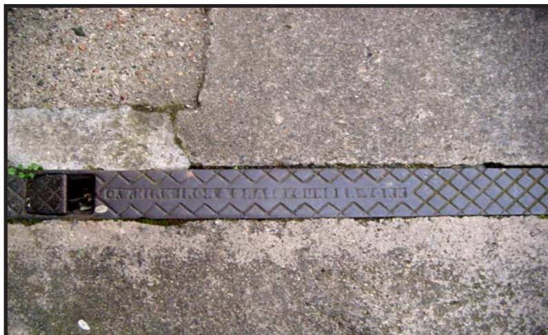
Example of drain cover in Leeman Road area
