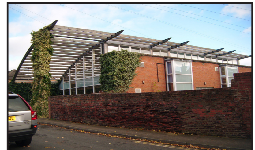
Late 20th century building at Highcliffe Court
