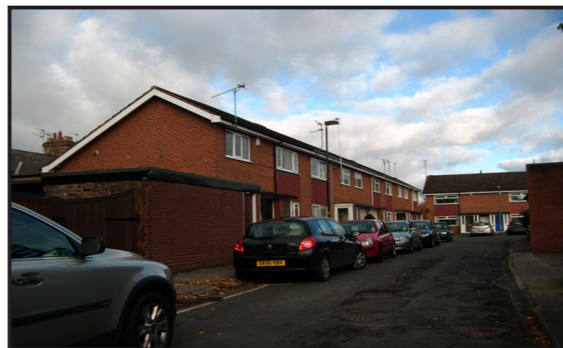
Mid to late 20th century housing at Highcliffe Court
