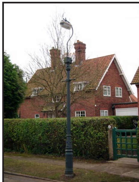
Above - Mid 20th century and modern street lighting on Galtres Grove Below- 1930s lighting on Rawcliffe Grove
