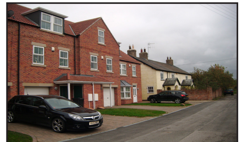
New builds and early 19th century cottage on Village Street
