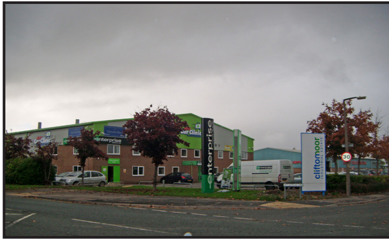
Industrial Estate buildings on Clifton Moor Gate
