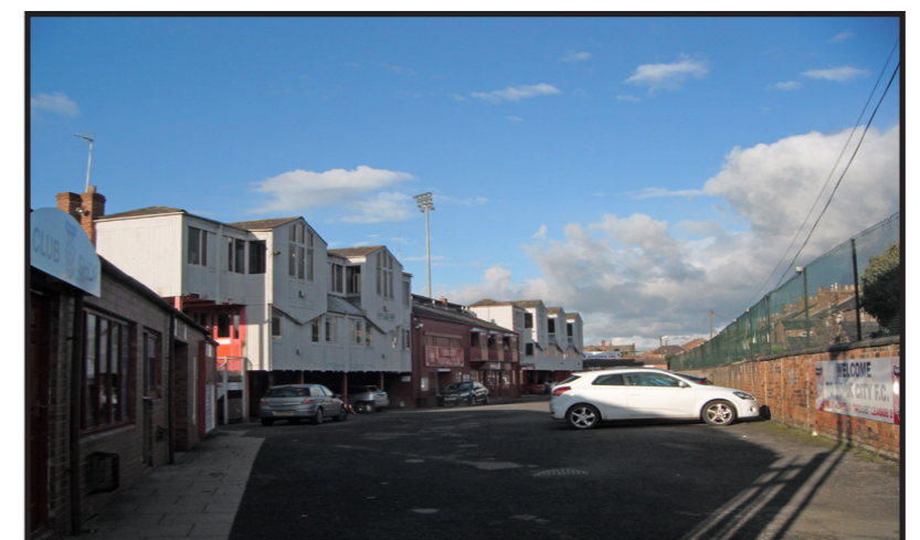
Bootham Crescent Football Ground
