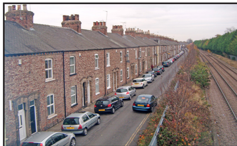
View of Filey Terrace from railway bridge
