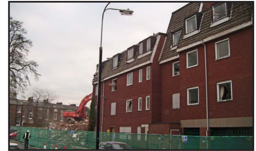
Demolition of Nurses Accommodation block 2013
