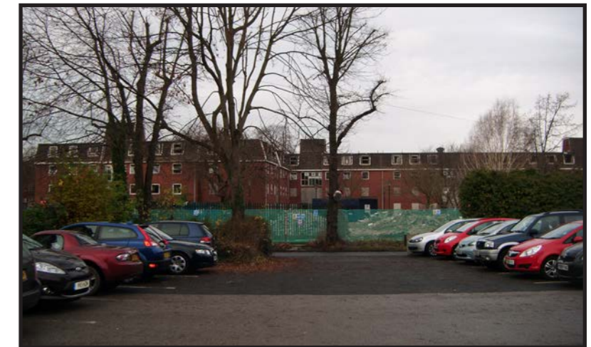
Rear of Nurses Accommodation Block during demolition
