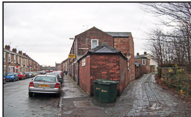
Kitchener Street front and rear showing stable pavours and historic signage
