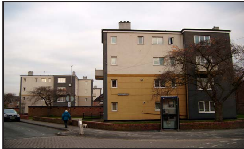
Re-faced 1960s flats on March Street
