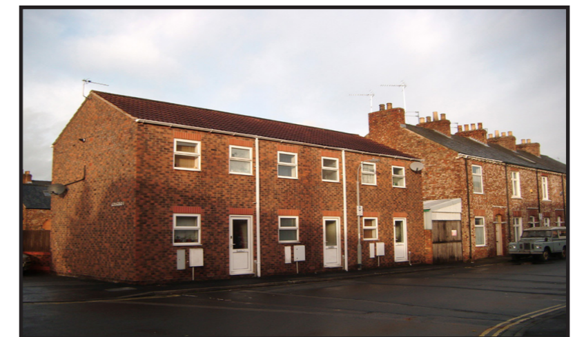
New builds constructed alongside 19th century buildings on Scaife Street
