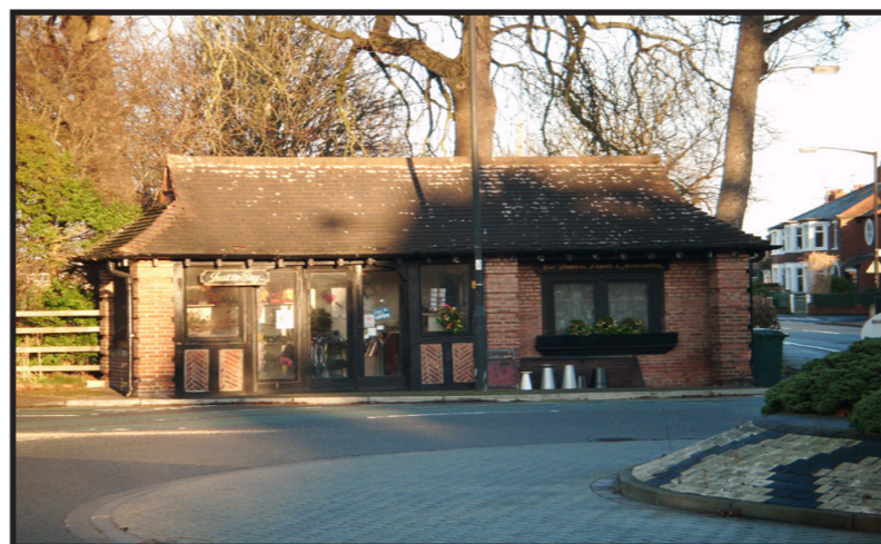
Former battery charging point, Heworth Green
