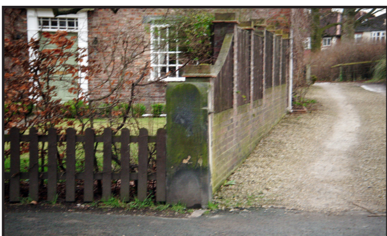
Remains of gate pier to Heworth Hall, Heworth village
