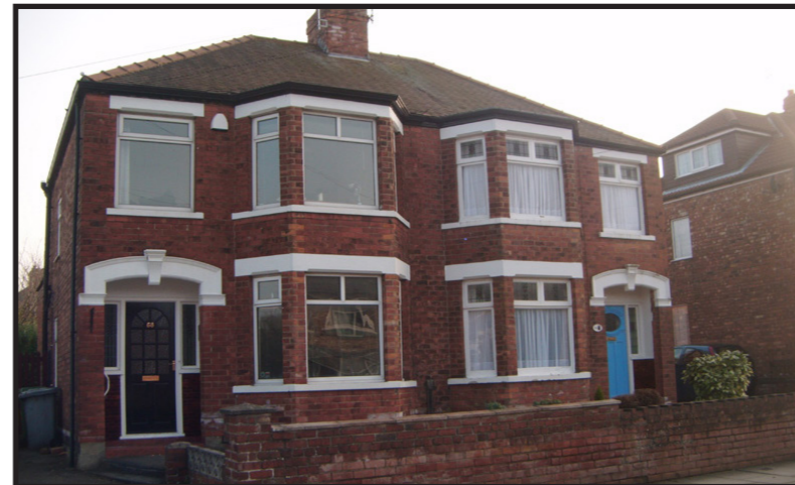
Example from Millfield Lane, note original style door (blue)
