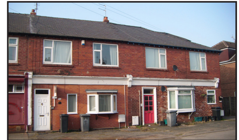
Former commercial buildings converted back into dwellings on Millfield Lane.
