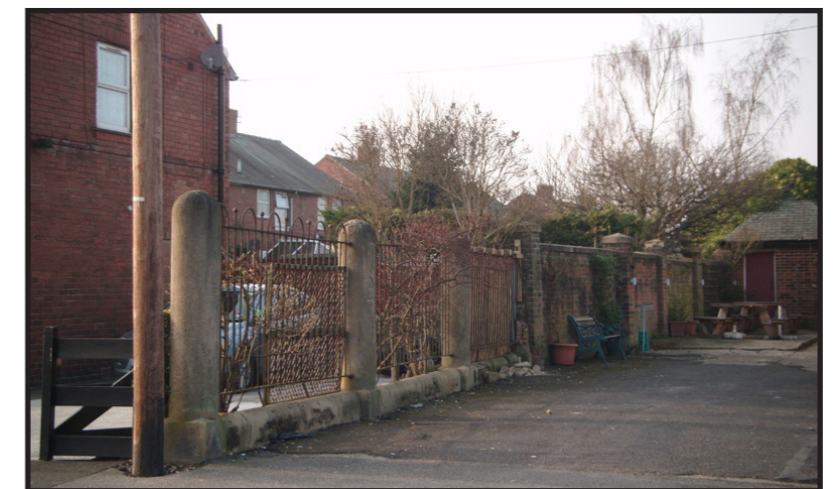
Concrete and iron walling in Magnet car park
