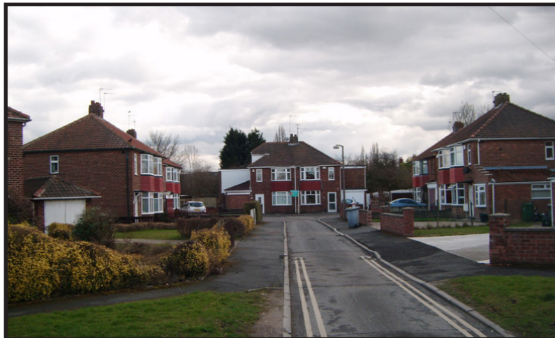
Gillamoor Avenue - house in background shows extensions either side and into loft space
