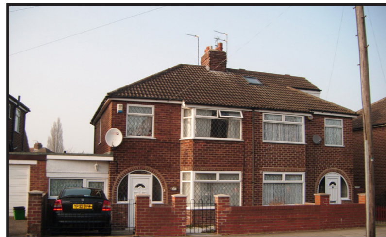
Example from Millfield Lane, note alterations to building e.g. infilled porch, garage and loft extension
