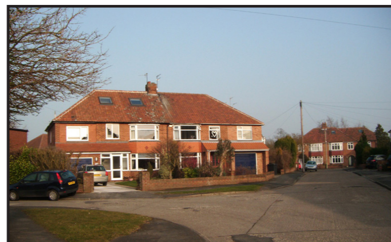
Moatfields housing showing concrete road surface and extensions to buildings.
