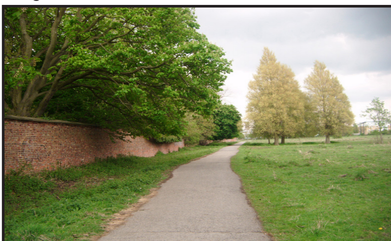
Asphalt path running alongside boundary wall taken from the west.
