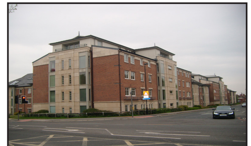
21st century flats on Hospital Fields Road.
