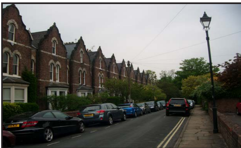
New Walk Terrace with period style lighting and Yorkstone paving
