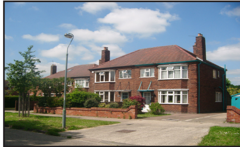
Example of housing on Broadway West,. Note the iron porch supports.
