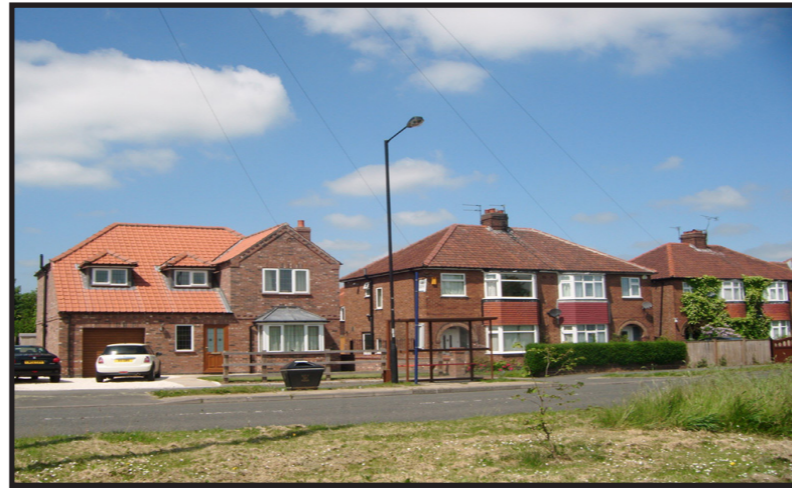
Heslington Lane showing original and new build housing
