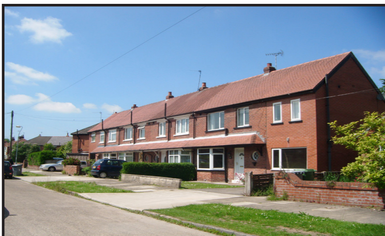
Lesley Avenue - note fenestration alterations and extension to right hand house
