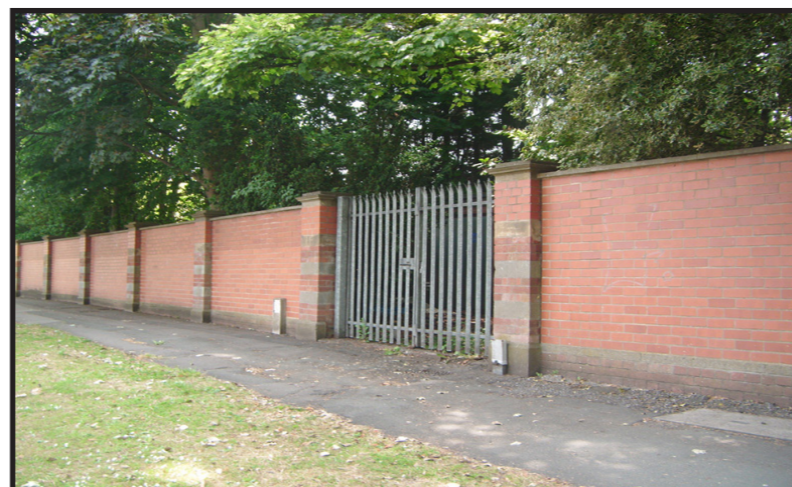
The boundary wall to Bishopthorpe Road.
