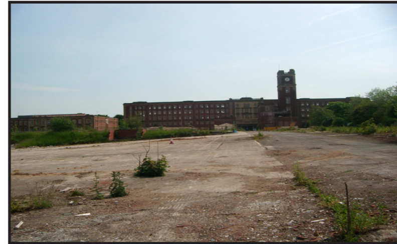
The Campleshon Road entrance following demolition to modern buildings.
