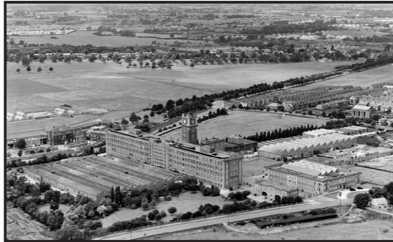
1950s aerial view of factory site - City of York Archives
