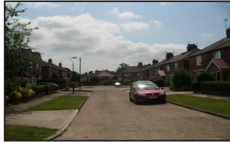
Finsbury Avenue with concrete road surface.
