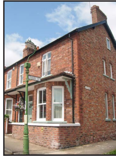
Terry Street showing historic street lighting.
