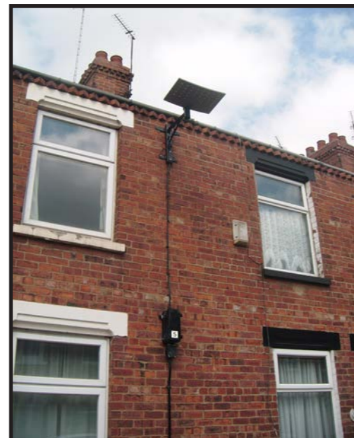
Early 21st century LED lantern attached to historic box on Queen Victoria Street (note also the loss of sash windows here)
