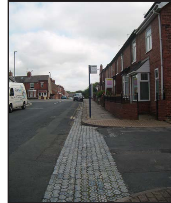
Stable paviour paving on Balmoral Terrace
