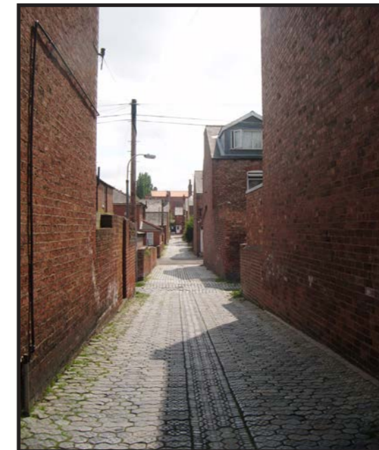
Stable paviour paving running N-S from South Bank Avenue to Jamieson Street.
