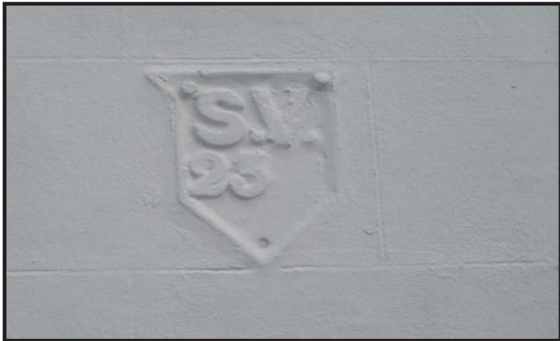
Painted over sluice valve marker on the side of the above shop.
