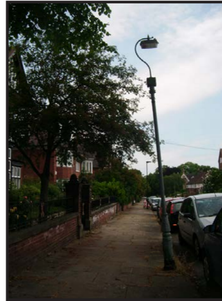
A leaning early street light on St. George's Place.
