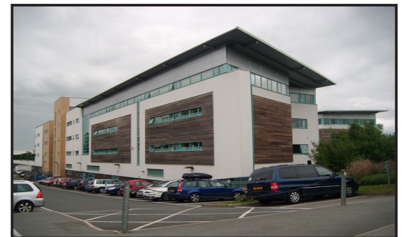
New college buildings
