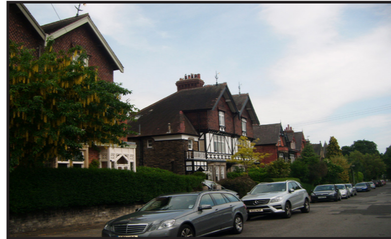
Housing on St. George's Place.
