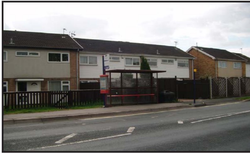
1980s social housing and streetscape components on Foxwood Lane.
