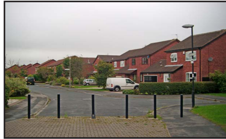
Examples of traditional 1980s brown frame windows and modern white replacements on Girvan Close.
