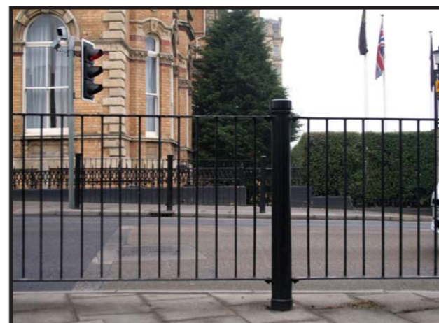
Simple and reasonably elegant railings on Station Road.
