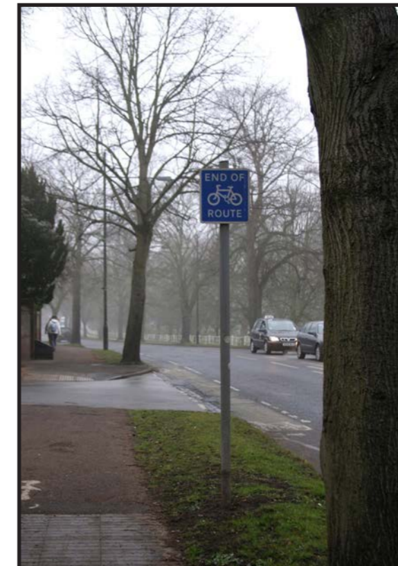
One of a pair of signs at a bus stop on Tadcaster Road that relate to an off road track meeting a main road but are poorly placed. City of York Standards & Principles for Designing Cycling Infrastructure should be followed.
