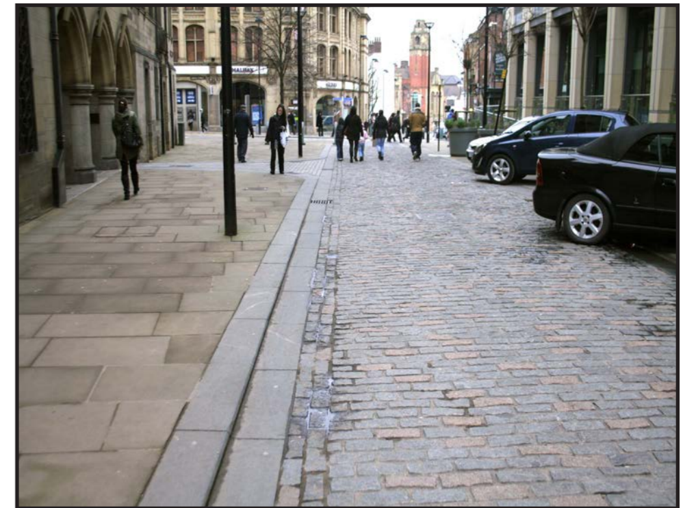
Good simple design in Sheffield using a small pallet of natural stone materials, in this case, granite setts on the carriageway, wide top granite kerbs and Marshall's Cromwell sandstone flags.
