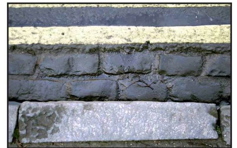
Brick drainage channel and granite kerb with neatly laid asphalt.
