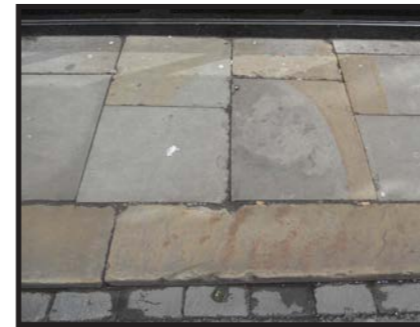
Diamond sawn English Pennine sandstone flags in Aldwark with a broad-top English Pennine sandstone kerb. Also note the blue/grey brick drainage channel
