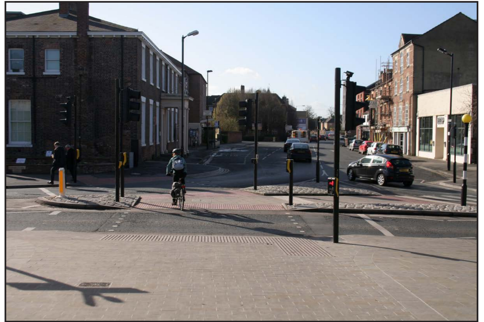
The recently (2013) re-designed crossing at the junction of Paragon Street and Fawset Street demonstrating significant improvement in cycle and pedestrian experience on the inner ring road.
