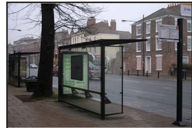
The right shelter but positioned incorrectly
