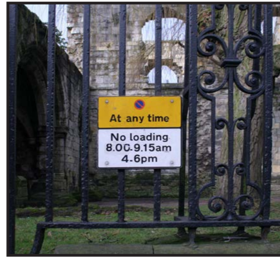
Sign fixed to listed railings detracting from historic setting and impacting on the railings.
