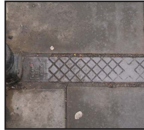
Two types of cast iron feature - on the left, an inspection cover by Dove and Sons, and on the right a cross footway rainwater channel by William Kirk.
