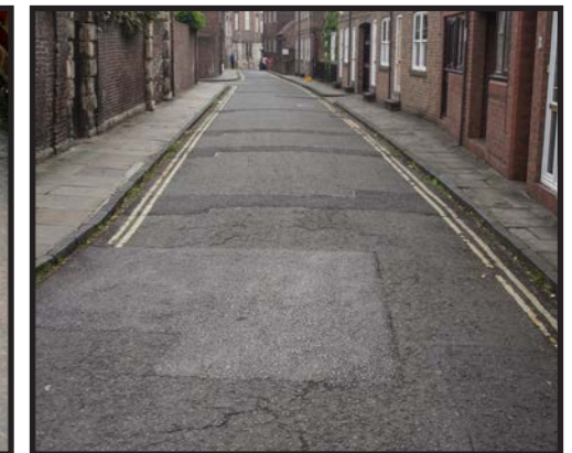
Asphalt carriageway surface in Aldwark with mixed aggregate inclusions providing an attractive variant to more ubiquitous plain asphalt surfacing
