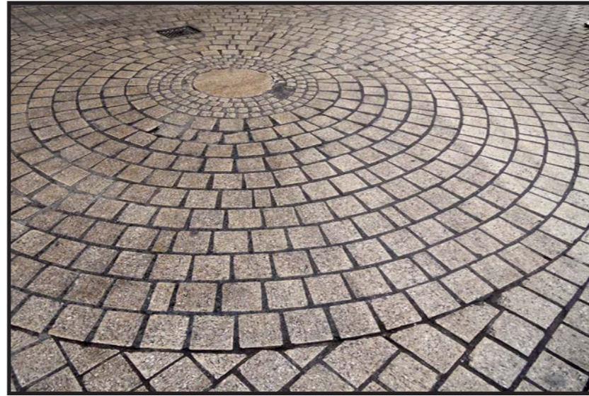
A fine example of the decorative use of blanc-de-bierge setts in Spurrriergate
