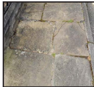
Traditional riven English Pennine sandstone flags in Bishophill. Note in this case the kerb is concrete.
