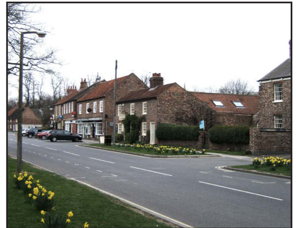
Heslington conservation area with grass verges, narrow pavements and parking outside shops. Note the concrete street light column
