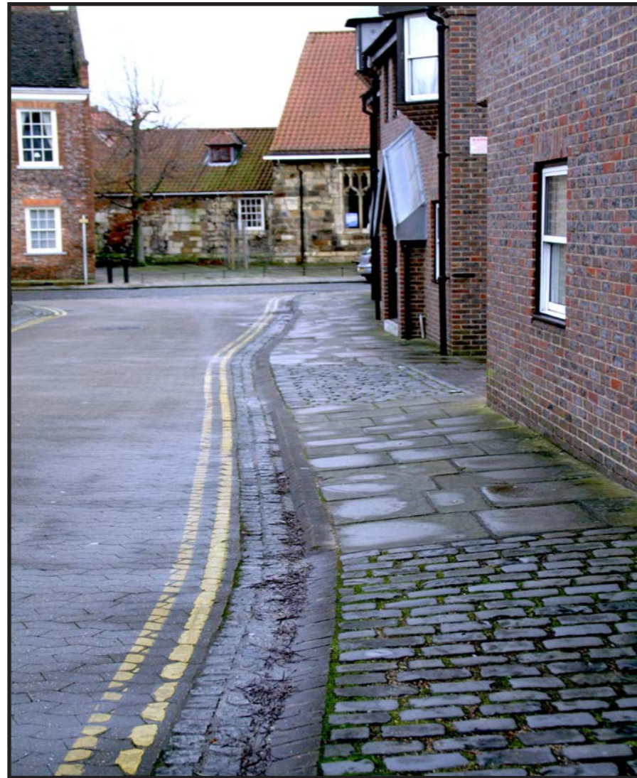
An example of the harmonious use of natural and contemporary materials in Aldwark, well laid and has lasted well
