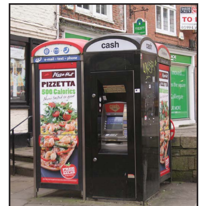
Group of modern kiosks in King's Square used as cash dispensers and telephones as well as unsightly street advertising. These are poor quality additions to the square
