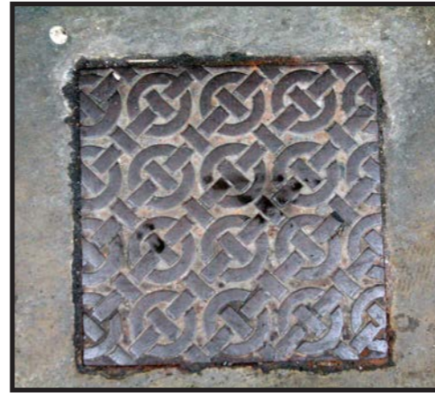
Two types of cast iron feature - on the left, an inspection cover by Dove and Sons, and on the right a cross footway rainwater channel by William Kirk.
