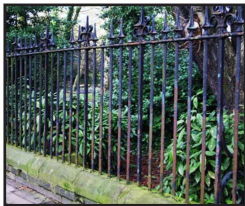
Listed railings at Bootham Hospital
