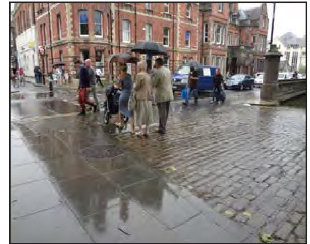
This exemplary raised crossing on Museum Street should be used as a model for other side road crossings in the city centre.
