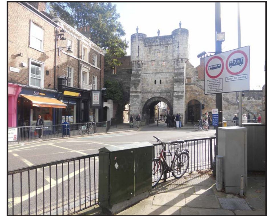
Railings at Bootham Bar - poor quality and combining with too many utility boxes significantly impacting on the setting of this important gateway into the city
