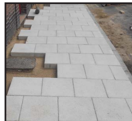
Grey Saxon paving in the process of being laid on Priory Street as a stretcher bond
