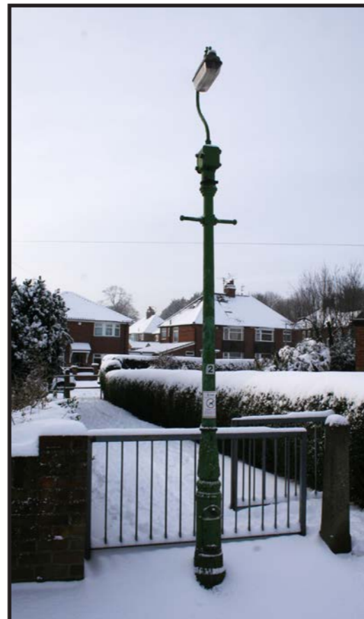
Street light from the 1950s with an attractive traditional swan neck fitting on Finsbury Avenue, off Bishopthorpe Road.
