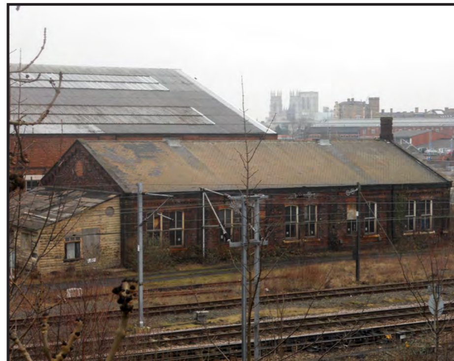
19th century engine shed that survived until 2012 when it was demolished for health & safety reasons
