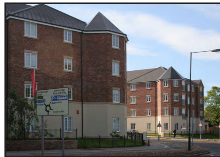
Four story apartment blocks on the old York College Site completely out of character to this part of suburban York in terms of massing height and design
