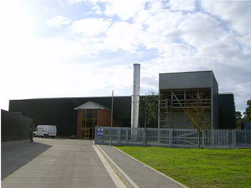
Eccleshall Biomass Power Plant - 2.6MW (Online Image) http://talbottpower.co.uk/
