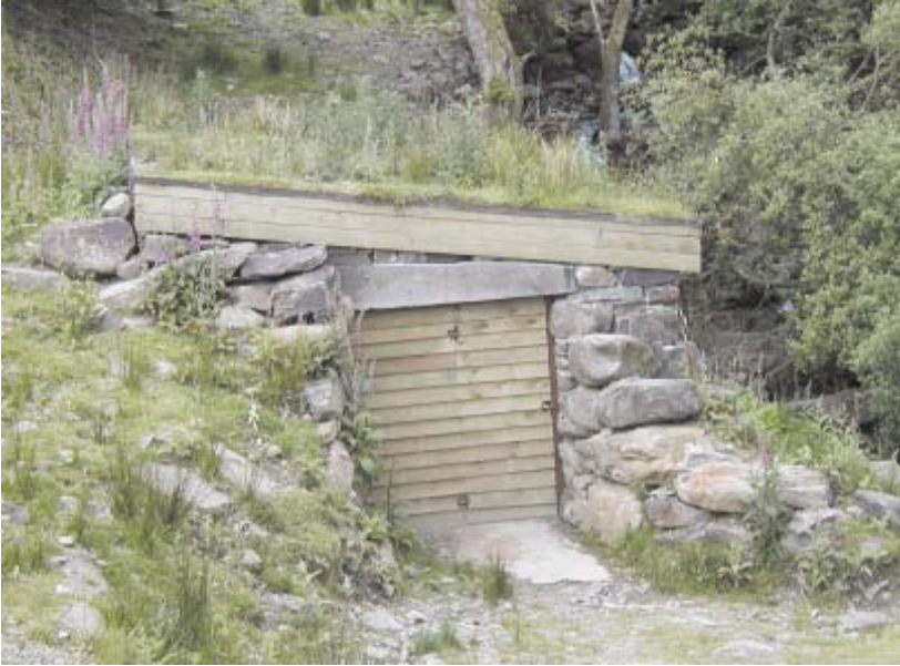
Turbine house for a 100kW hydro plant. Taken from Planning for Renewable Energy: A Companion Guide to PPS22 (OPDM), 2004
