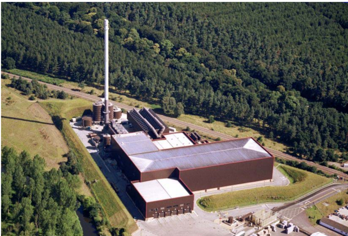
Thetford Biomass Power Station - 38.5MW (Online Image) http://www1e.btwebworld.com/fibrowatt/UK-Thetford/index.html
