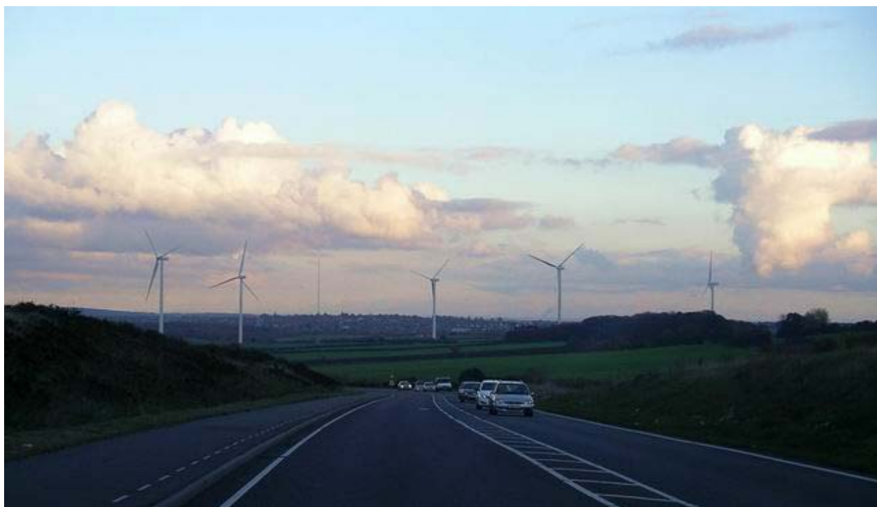
Lyndhurst Wind Farm, Nottingham (Online Image) © Copyright Lynne Kirton and licensed for reuse under this Creative Commons Licence .
