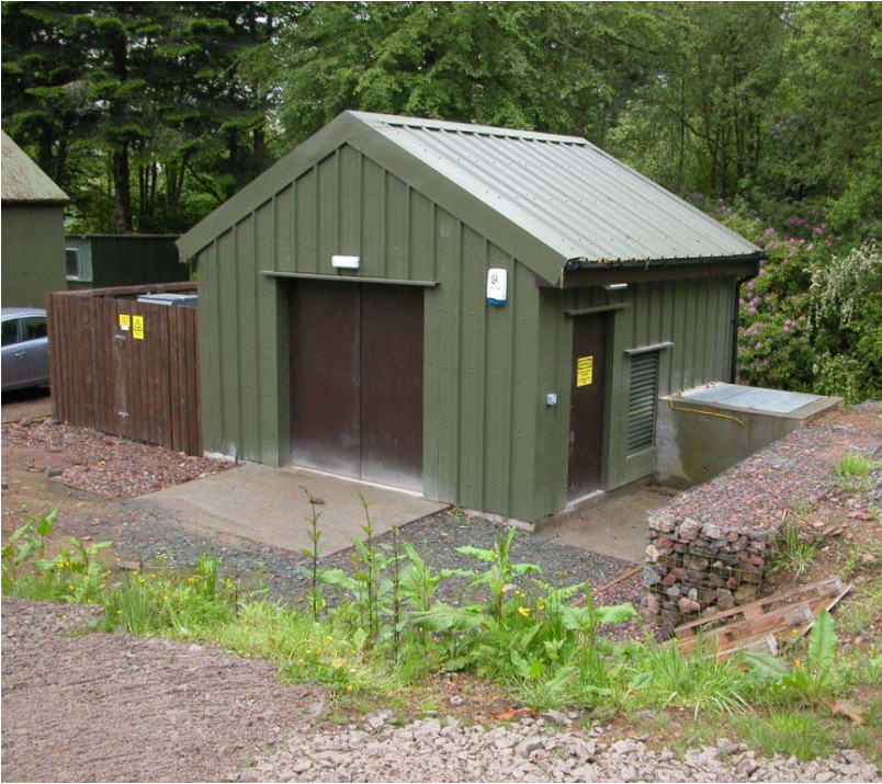
Example of metal clad turbine house, N Buchan.
