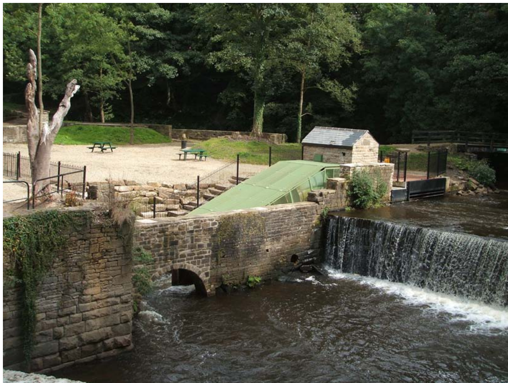
Archimedes screw and turbine house of stone construction, Appleton
