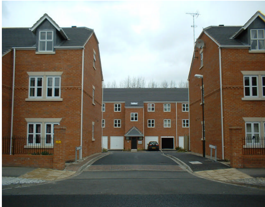
Figure 6 – Access to apartment blocks
