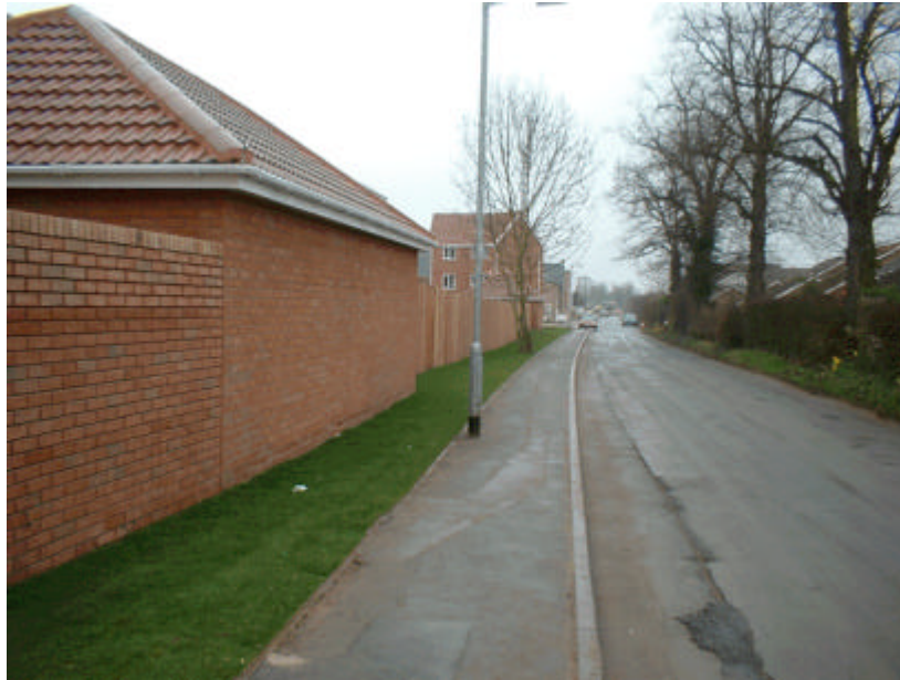
Figure 5 – A service verge
