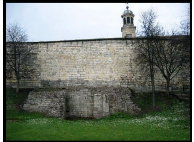
Figure 4 Curtain wall and remnants of the south gate
