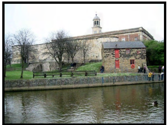
Figure 14 The Castle as seen from Castle Mills Bridge
