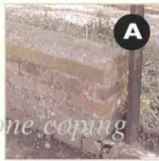
Walls with limestone coping
