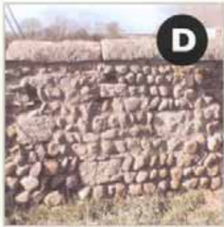
Wall and brick texture and colour
