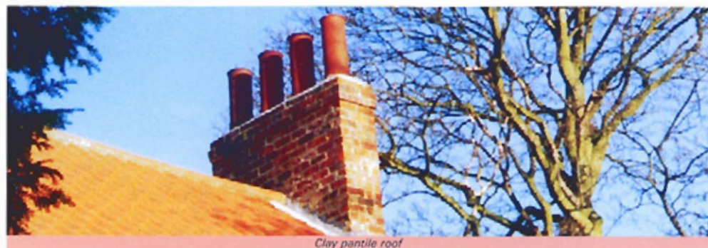
Clay pantile roof
