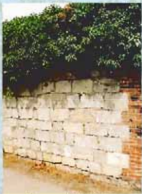
Stone wall, Main Street
