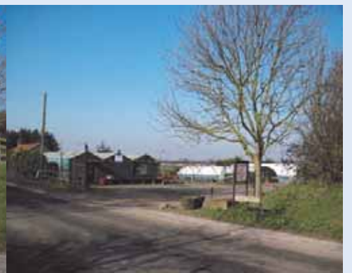
Disused nursery buildings.
