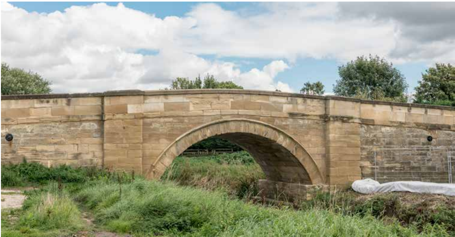
Strensall Bridge: John Carr’s bridge
