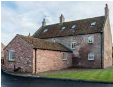
Low Farmhouse – Towthorpe Road
