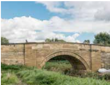
Strensall Bridge – Sheriff Hutton Road
