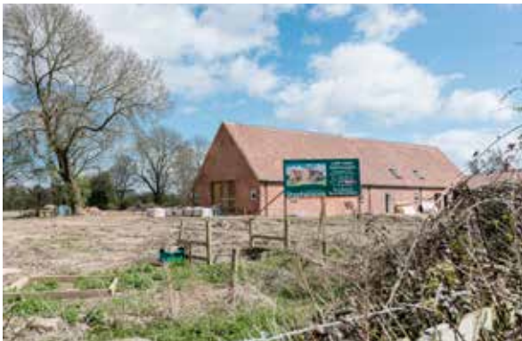
Towthorpe: conversion of agricultural buildings
