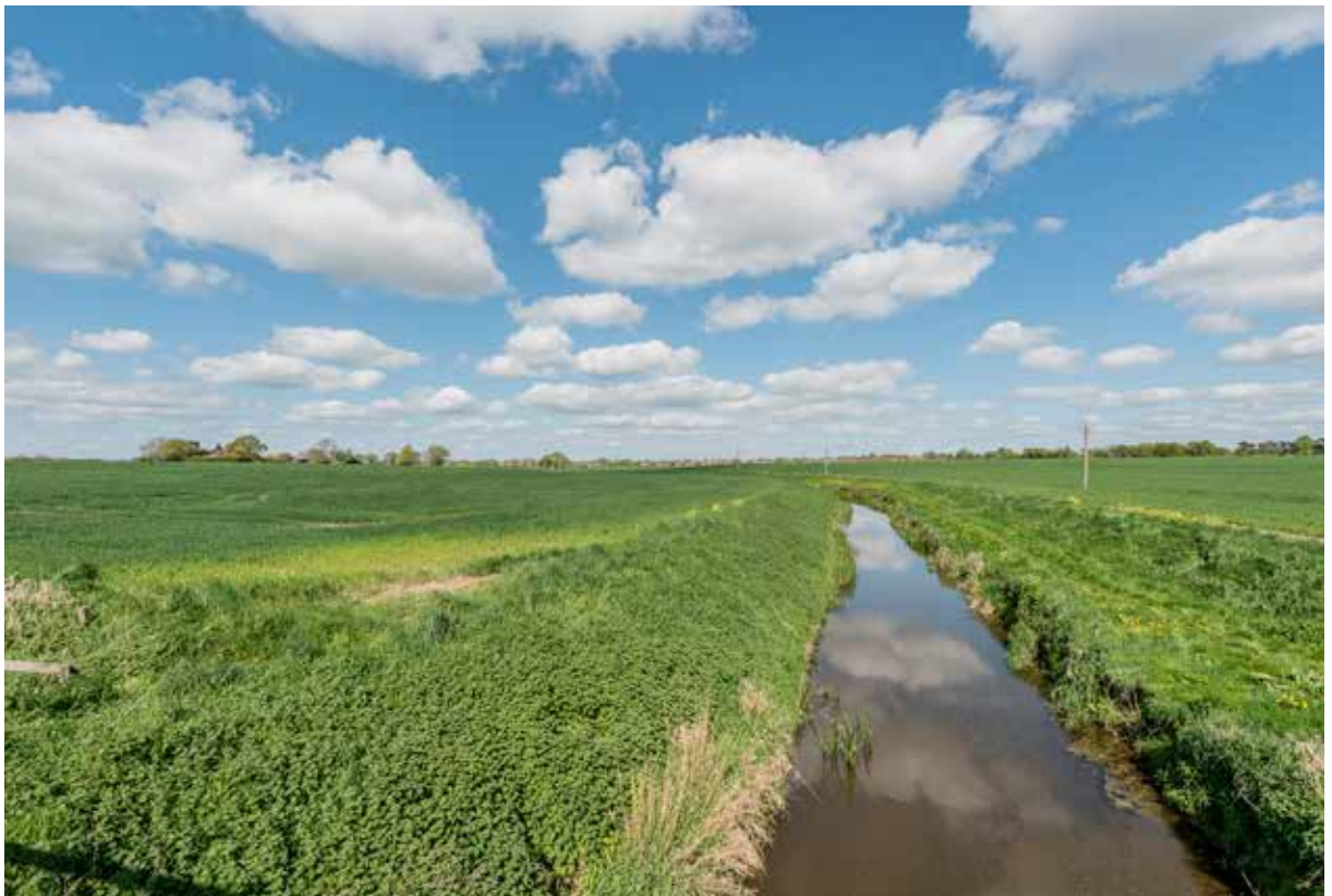
a2. Northeast from Towthorpe Bridge
