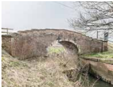
Strensall New Bridge – Haxby Moor Road
