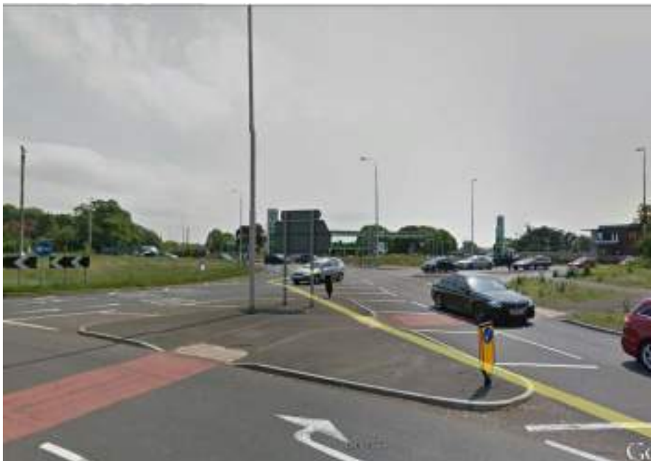
Figure 5.5 – Road site facilities on the A1237
