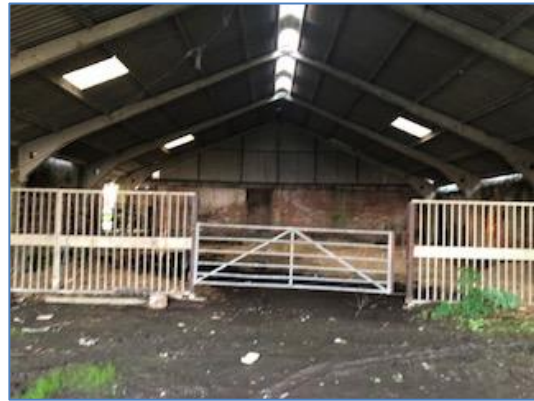
Photo 36: Building 8, entrance to fold yard.
