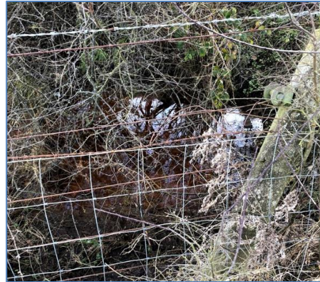
Photo 14: TN 17, overgrown ditch
