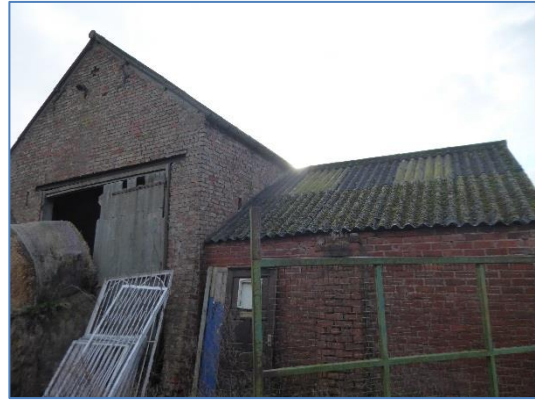
Photo 28: Building 4 external, and the gable of Building 7
