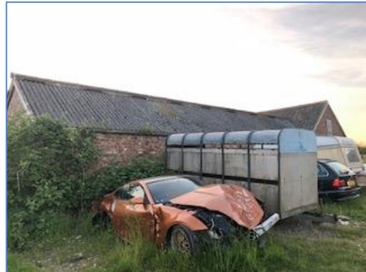
Photo 38: Building 10, eastern aspect
