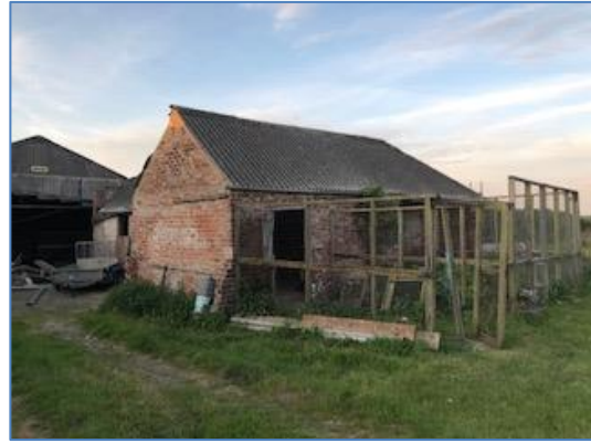
Photo 40: Building 12. Southern aspect
