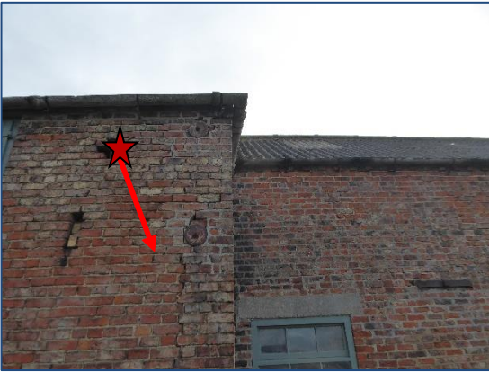
Photo 56: Building 7, vent in western wall
