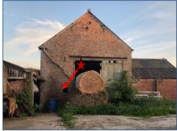
Photo 55: Building 7, northern open barn door
