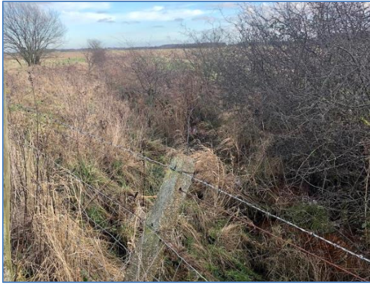
Photo 13: TN 17, overgrown ditch
