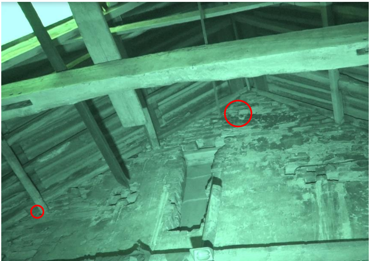
Photo 58: Emergence location inside building 7
