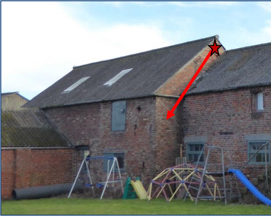
Photo 54: Building 7, southern gable end
