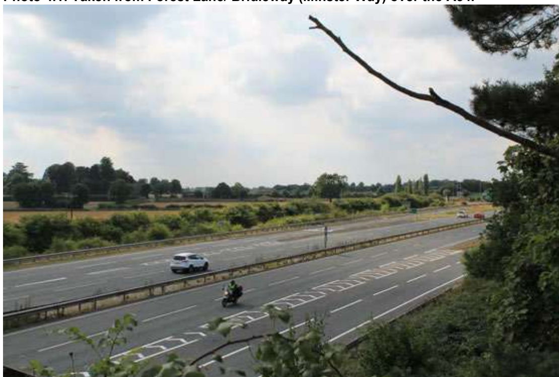
Photo 4.1: Taken from Forest Lane/ Bridleway (Minster Way) over the A64.
