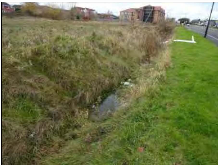
Photograph 7 showing the ditch
