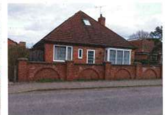
8. Existing residential dwellings on Moor Lane
