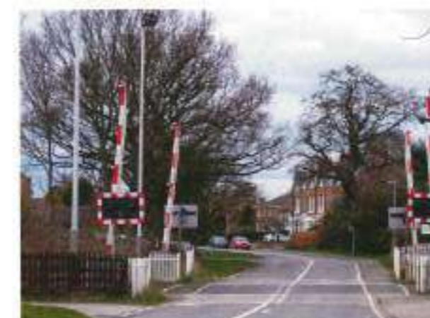
7. Railway crossing on Moor Road
