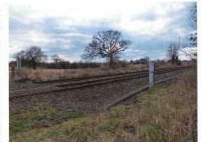
6. Railway Line dissecting the site east west
