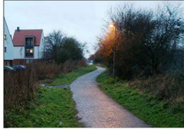
(segregated route near Derwenthorpe)
