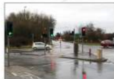
Pedestrian and cycle facilities at Osbalwick Link Road junction
