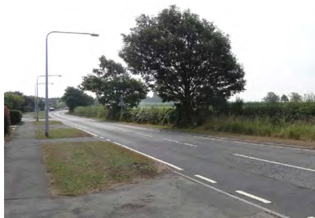
Figure 12: Looking South on Manor Heath
