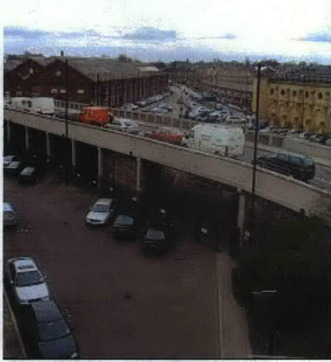
Figure 18 - Queen Street Bridge, Towards Station Car Park
