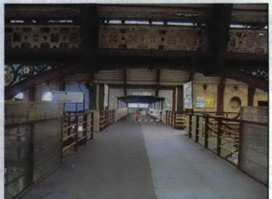
Figure 17 - York Station Main Footbridge, with Extension to Platforms 10/11 in Background
