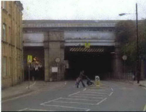
Figure 12 - Marble Arch / Leeman Road Tunnel, Eastern Portal
