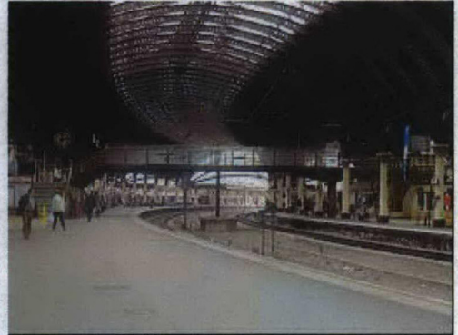
Figure 16 - York Station Footbridge
