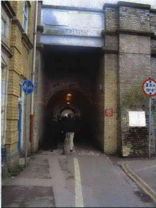
Figure 13 - Marble Arch Foot Tunnel, Eastern Portal
