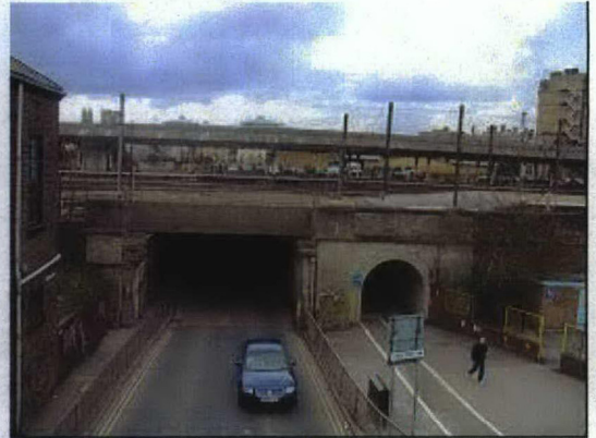
Figure 15 - Marble Arch / Leeman Road Tunnel, Western Portal
