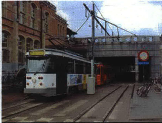
Figure 27 - Ghent Railway Station - Tram Tunnel
