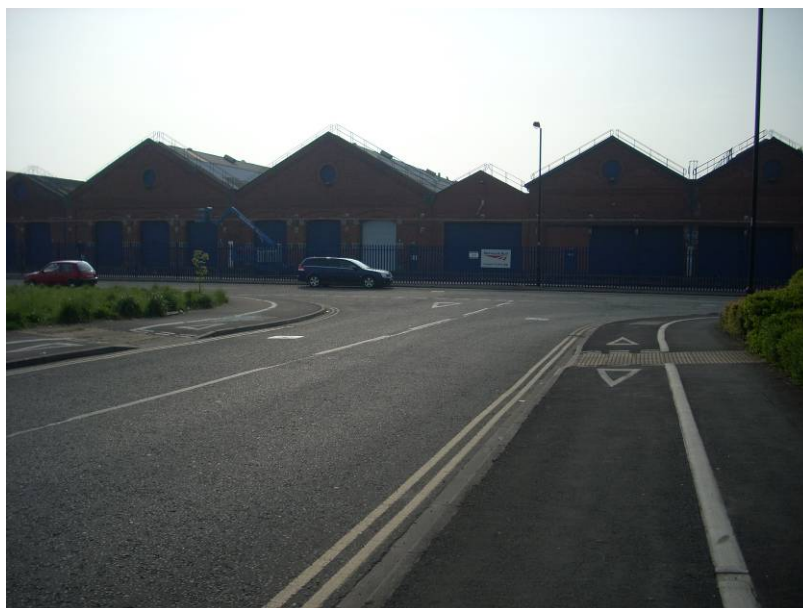
Plate 5.4 Existing Priority Junction at the eastern end of Holgate Park Drive with the Thrall works in the background
