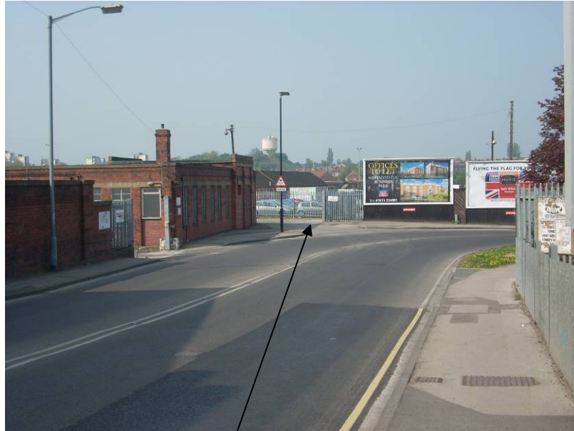
Plate 7.1 View from Leeman Road showing possible access point at existing Network Rail entrance
