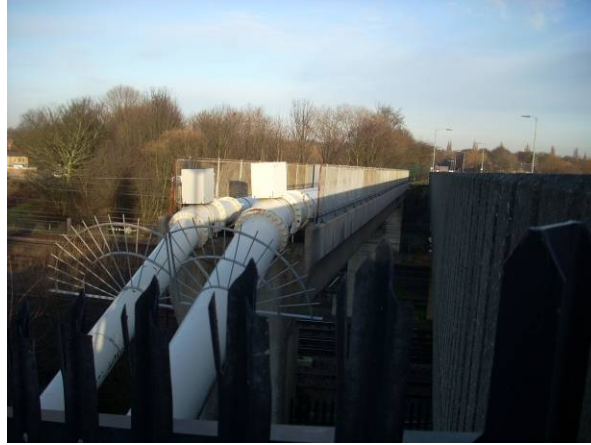
Plate 6.1 Pipe Bridge on the northern side of Severus Bridge
