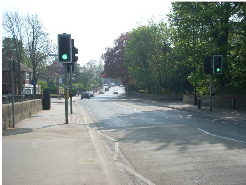
Plate 4.1 Existing Priority Crossroads at the Chancery Rise/Holgate Road junction
