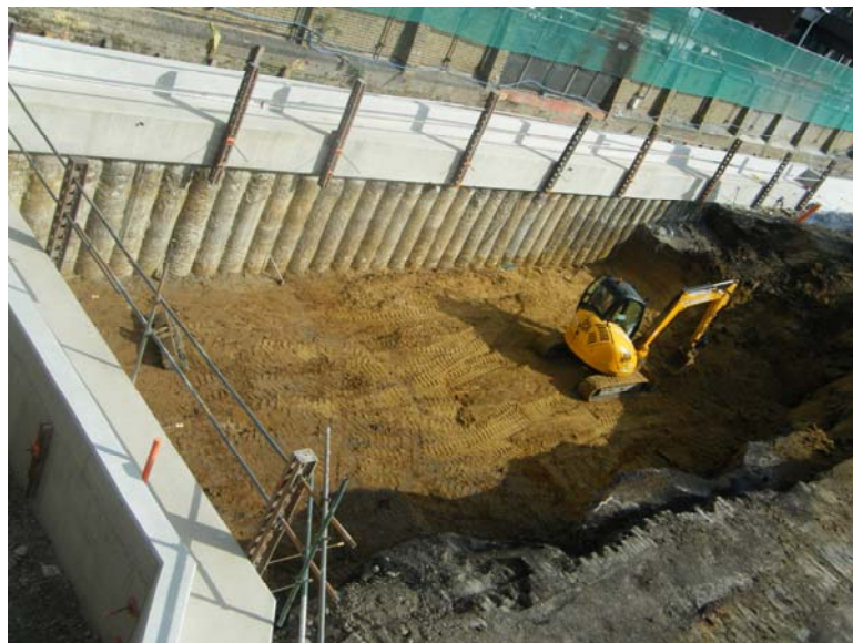
Plate 8.3 Secant Pile Wall (Paddington Station, London)
