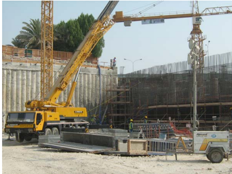
Plate 8.3 Secant Pile Wall (Paddington Station, London)
