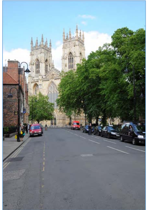
Image 15 – View from Duncombe Place towards the Minster.
