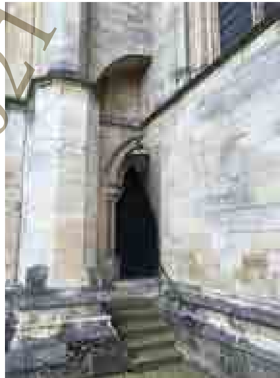
Fig. 11: 'Hidden door' in west elevation
