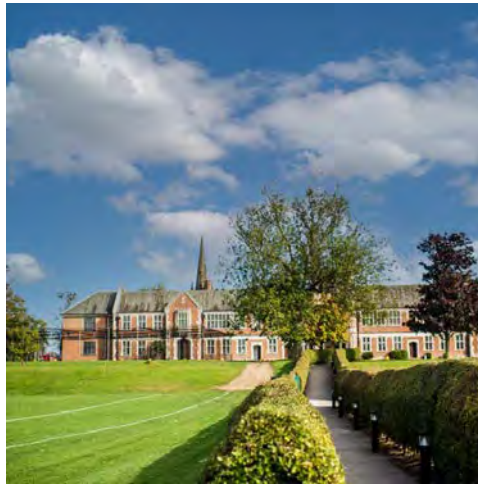
Footpath linking Queens Building with swimming pool
