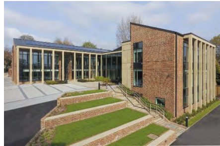
Pascal Building, north campus
