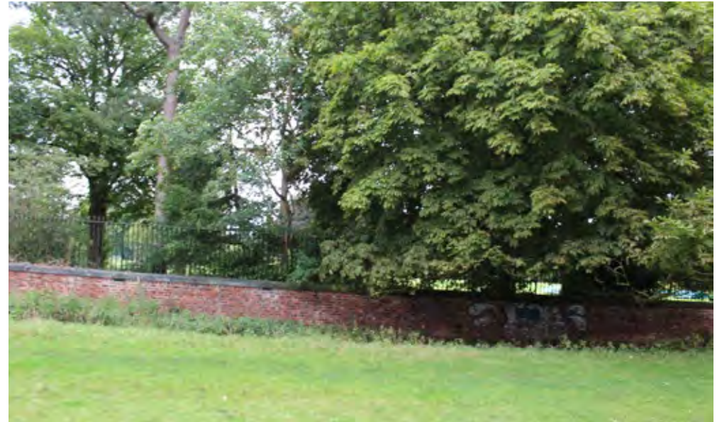
▲ E. The high brick wall along the western edge reduces in height and is replaced with railings for a portion of the boundary before returning to a high wall.
