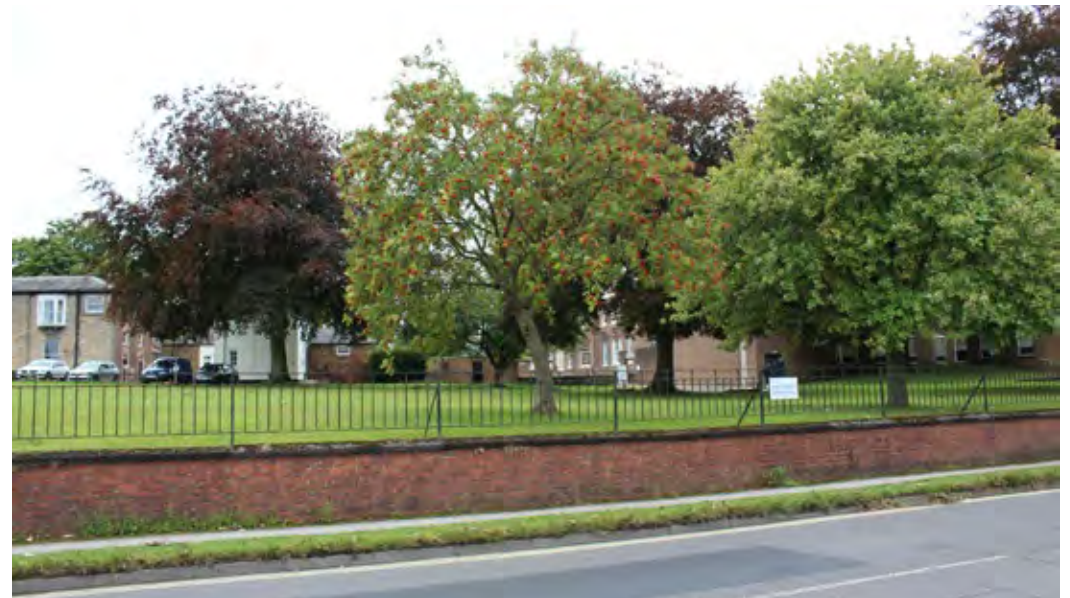
▲ B. Brick retaining wall with metal railings adjacent to Heslington Road near the entrance to The Retreat.
