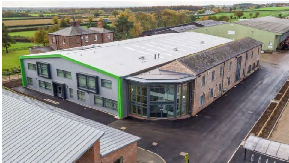
Lance Gilling Agri Tech Centre, completed 2018
