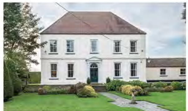
Manor House Farmhouse, Strensall
