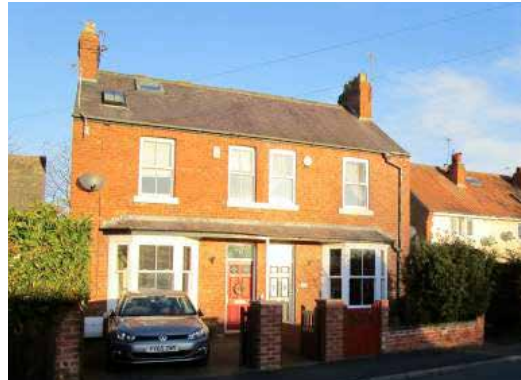
Photo 24: Example of nineteenth century semi-detached housing
