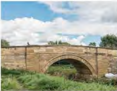
Strensall Bridge – Sheriff Hutton Road
