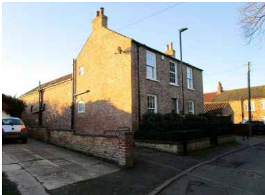
Photo 34: Example of detached house with rear wing
