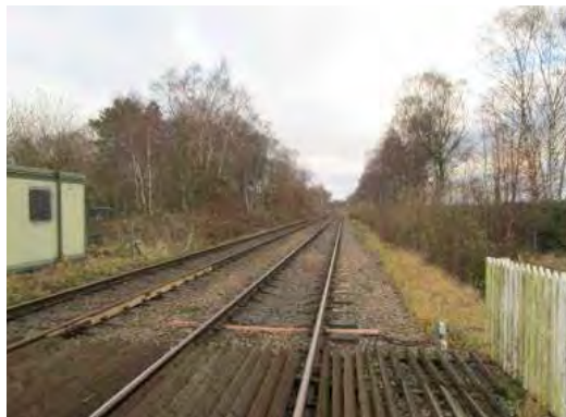
Photo 3: View of the railway line
