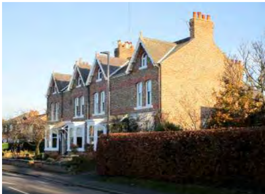
Photo 23: Terrace development with additional rooms accommodated within the roof space
