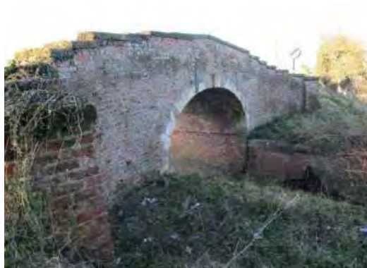
Photo 9: Strensall New Bridge
