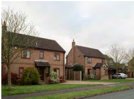
Photo 25: Twentieth century two storey housing
