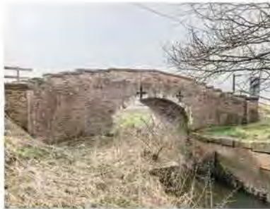
Strensall New Bridge – Haxby Moor Road
