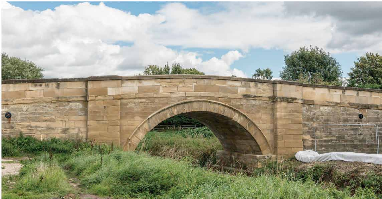
Strensall Bridge: John Carr’s bridge
