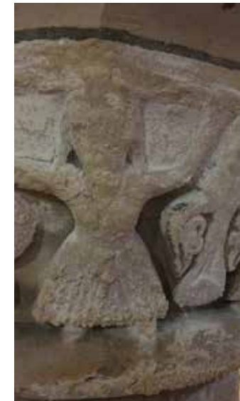
Stone corrosion
