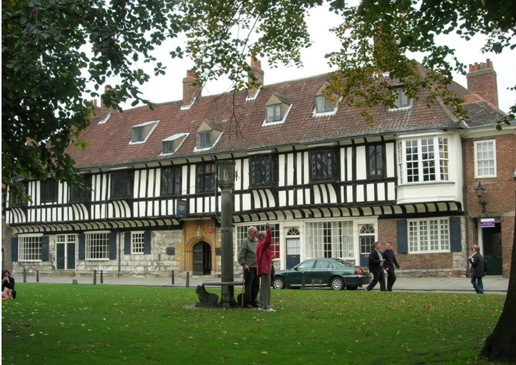
Illus. 5. St William's College, 1465: demonstrates conservation practice at the beginning of the twentieth-century
